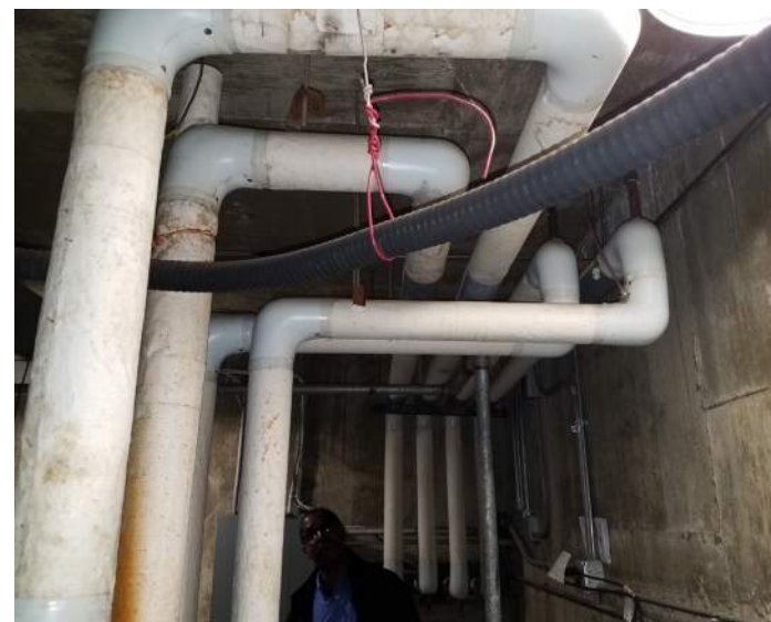
Typical condition of pipe insulation
