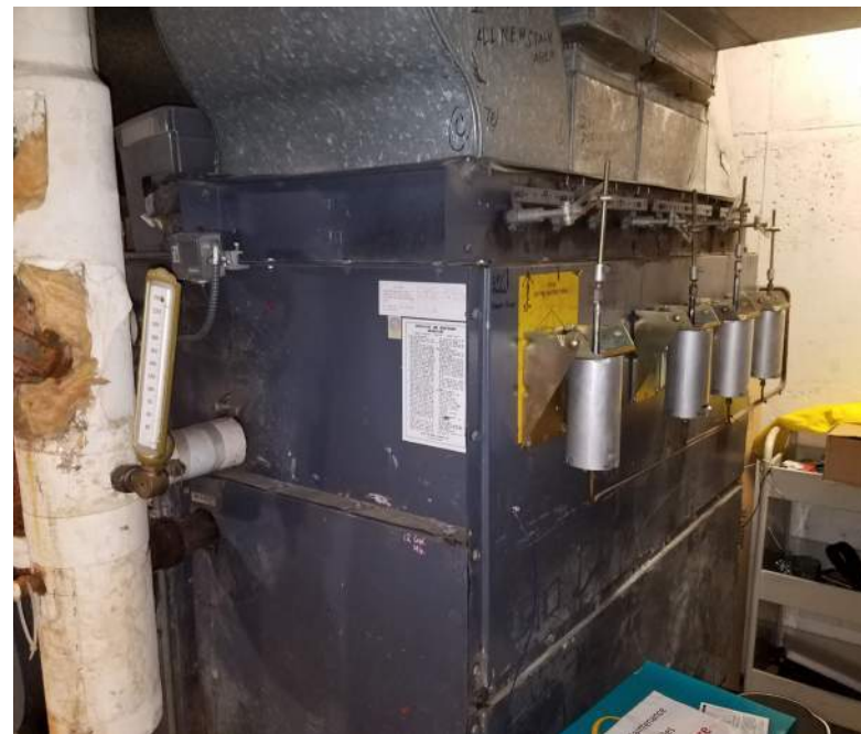
Multi-zone air handling unit with hot and chilled water piping connections.
