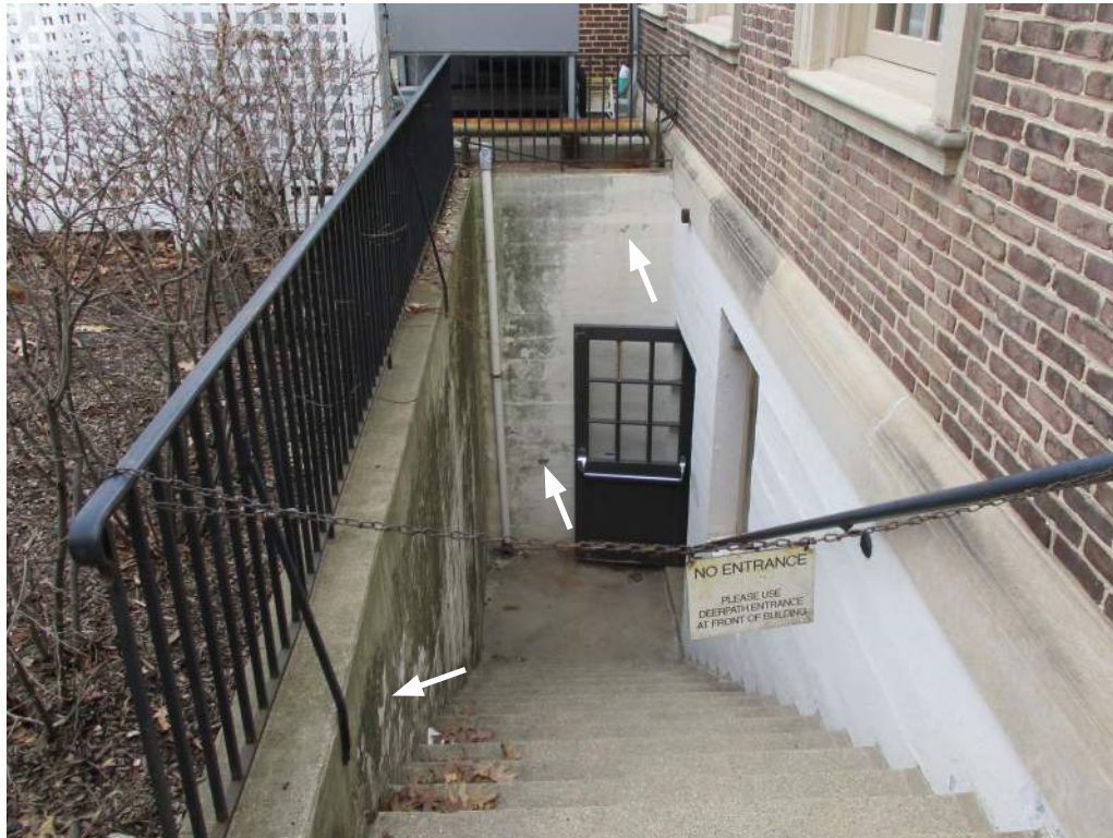
EXTERIOR STAIR (WEST)
