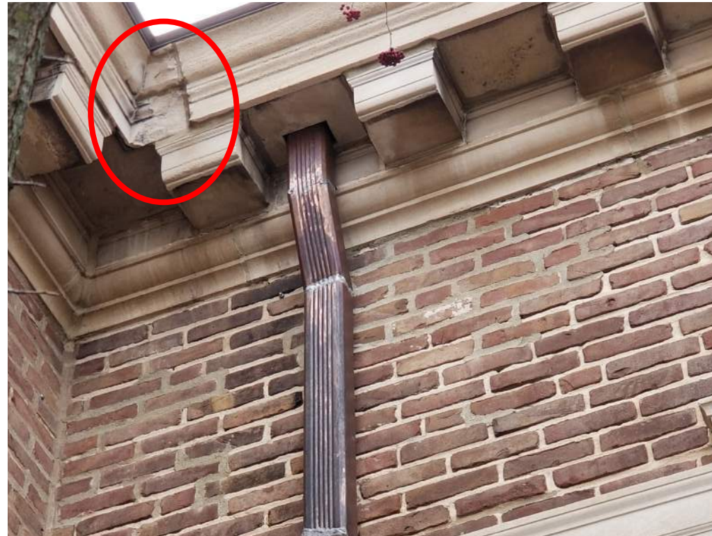
NORTH WING - WEST FACADE
