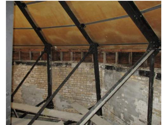
Steel trusses supporting dome
