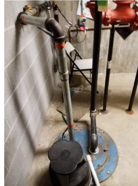
Typical sewage ejector
