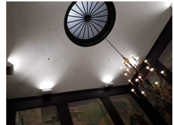
Central Rotunda Up-Lights
