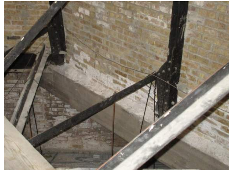
Current condition of the inside face of the dome pedestal observed from the attic space above the rotunda. Extensive efflorescence corresponds to locations near roof system transitions. Signs of prolonged water infiltration, including areas of heaviest accumulation of efflorescence, occurs adjacent to sloped corners.
