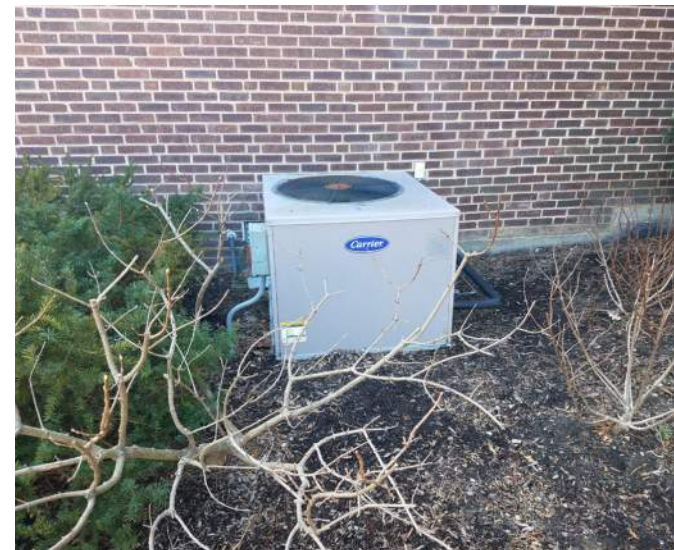
Smaller capacity air cooled condensing unit
