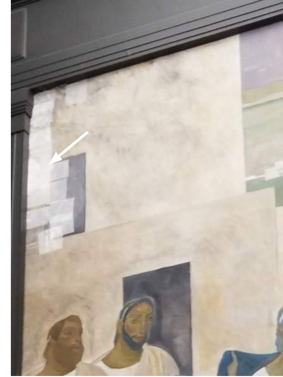
Panel III- patch repairs at upper (L) corner.
