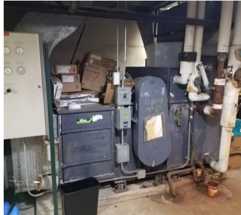
Multi-zone air handling unit with hot and chilled water piping connections.
