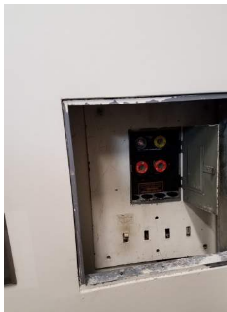
“Hidden” Fused Panel – Second Floor
