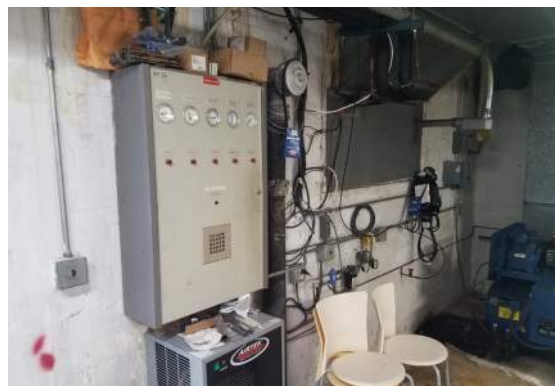
Typical pneumatic temperature control panel
