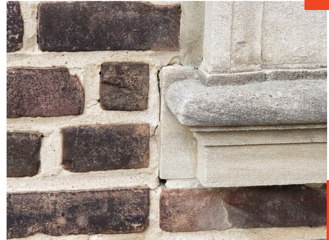
NORTH WING - WEST FACADE
