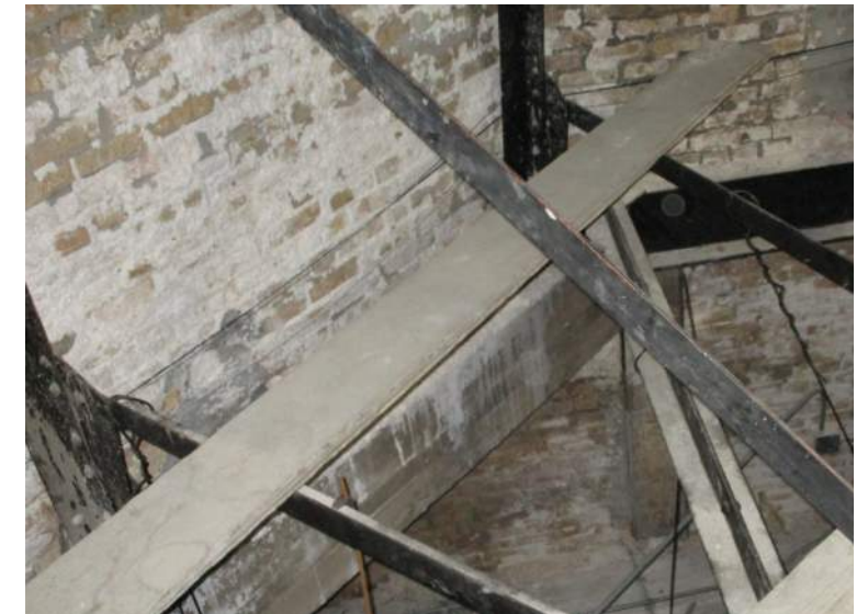
Current condition of the inside face of the dome pedestal observed from the attic space above the rotunda. Extensive efflorescence corresponds to locations near roof system transitions. Signs of prolonged water infiltration, including areas of heaviest accumulation of efflorescence, occurs adjacent to sloped corners.
