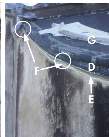
Typical copper roofing edge
