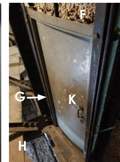
Door into plaster light shaft from attic
