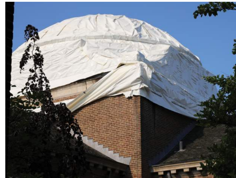
Temporary protection (July, 2018)
