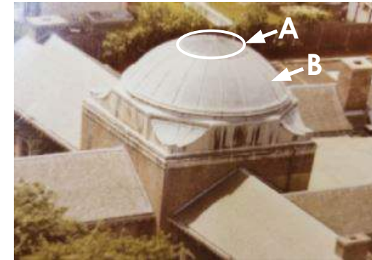
Skylight at top of dome
