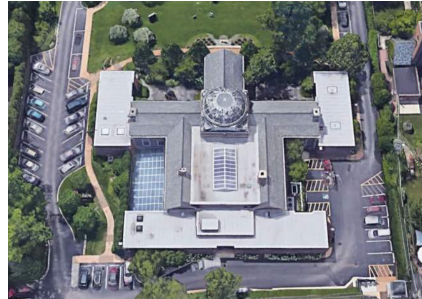
Aerial view - looking south
