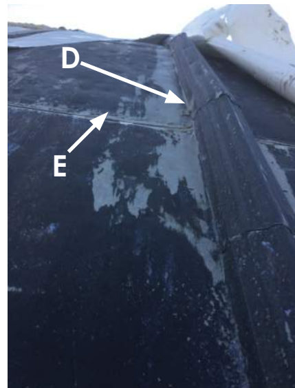
Dome roof pans and battens
