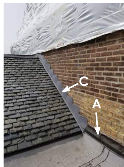
Flashings at east side of dome
