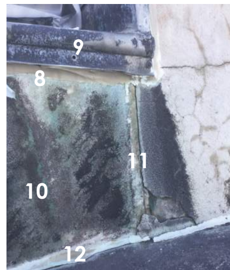
Stone joint at corner pier
