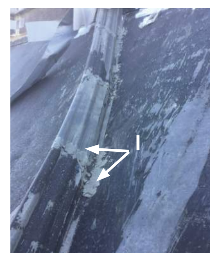
Typical batten on sloped corner roof copper
