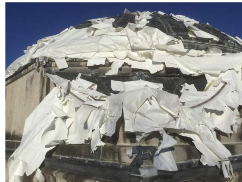
Temporary protection (December, 2018)
