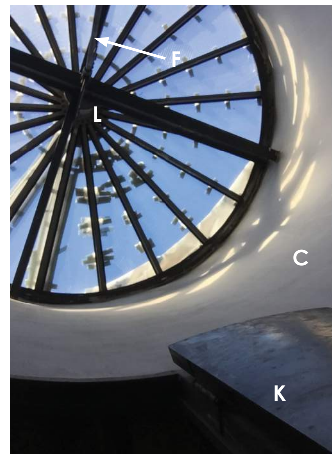
Skylight view from within light shaft
