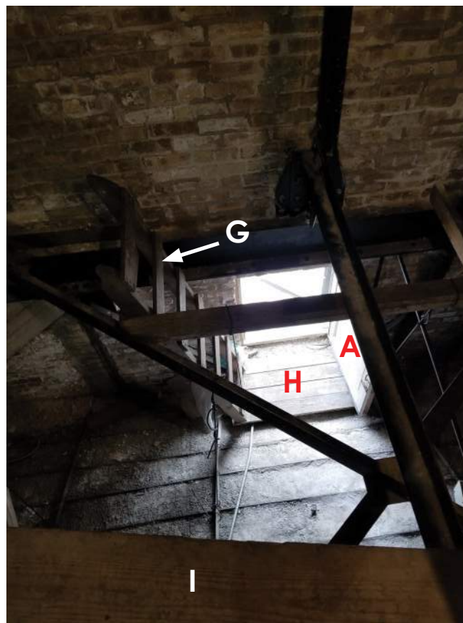
Inside attic looking down to exterior access door
