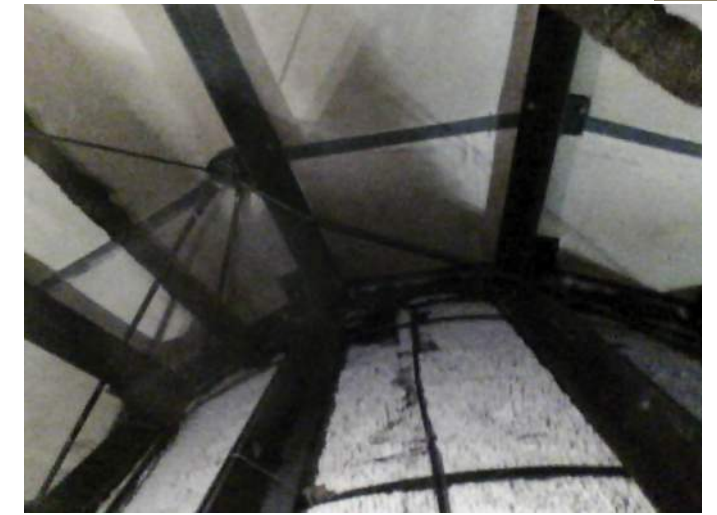
Infrared image and accompanying photo looking up at the juncture of the dome and the plaster light shaft in the attic. These images help to understand where potential water issues exist beyond what is visible to the eye.
