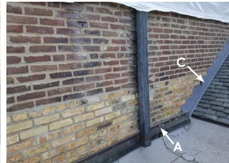
Flashings at west side of dome
