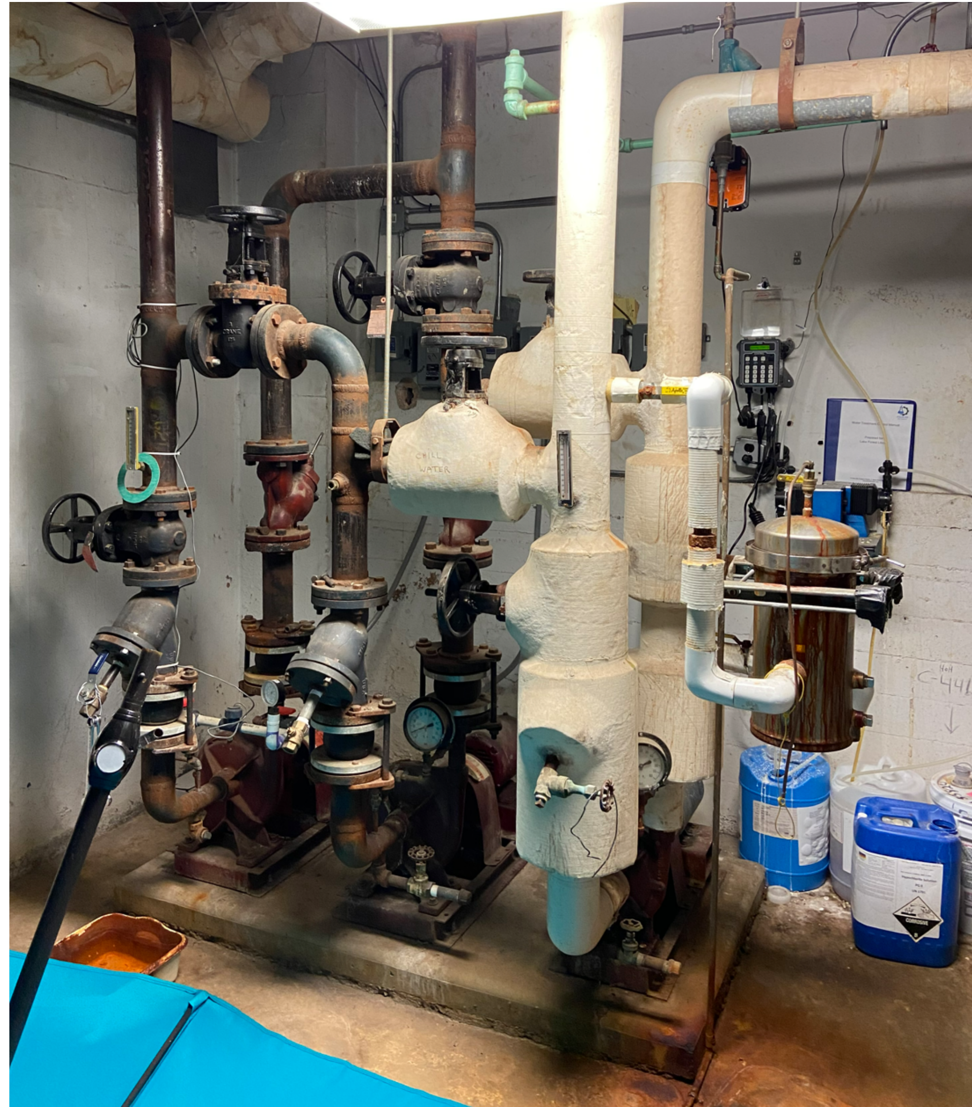
1. REMOVE EXISTING CHILLED WATER AND CONDENSER WATER PUMPS, PIPING, ELECTRICAL AND CONTROLS.
