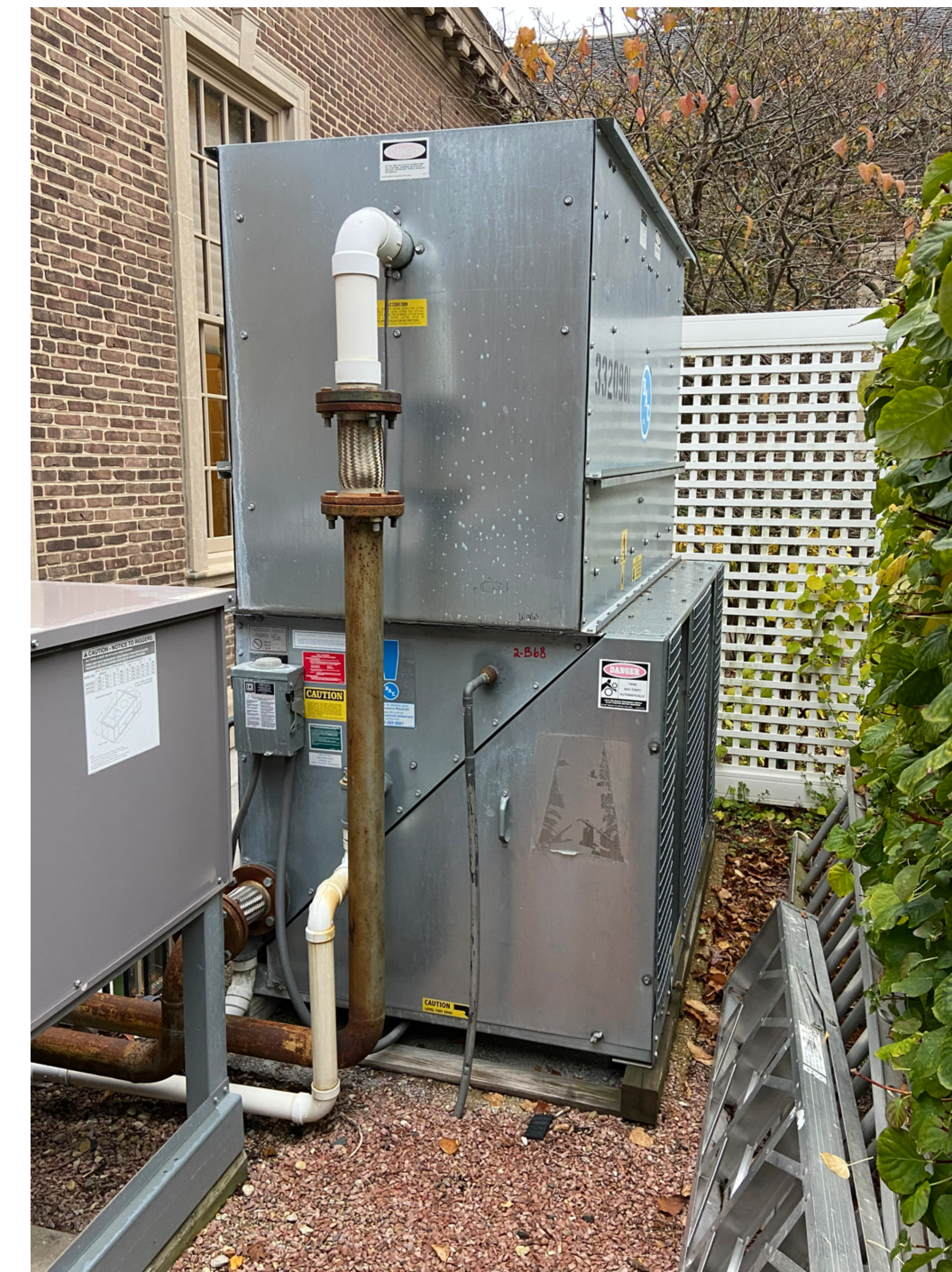
3. REMOVE EXISTING COOLING TOWER, PIPING, ELECTRICAL AND CONTROLS.
