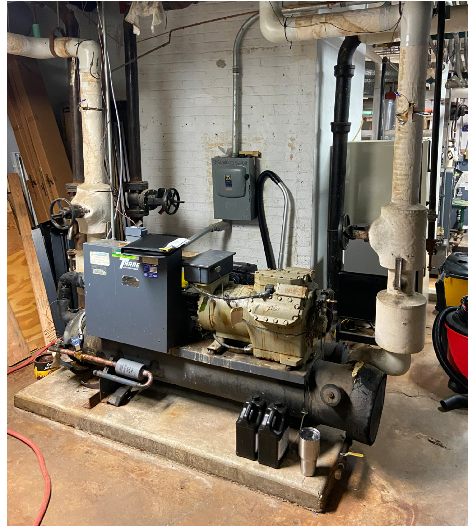
2. REMOVE EXISTING WATER COOLED CHILLER, PIPING, ELECTRICAL AND CONTROLS.
