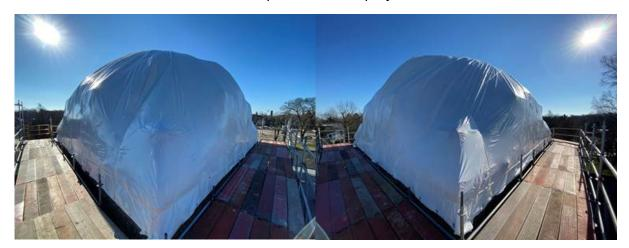
Extra shrink wrap heated and wrapped over sharp corners. This was an area where the previous wrap had started to give out. Belfor cut and adhered extra wrap here to help reduce the time in which the dome will break through the tarp.
